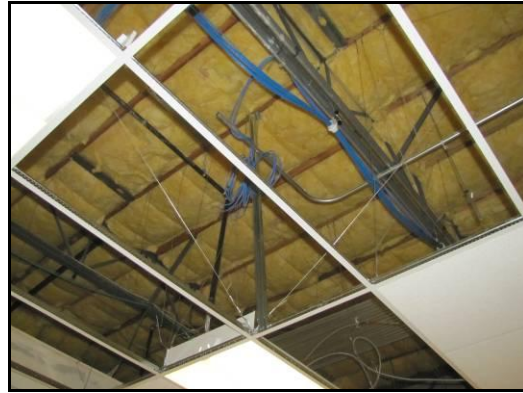
Bracing of suspended ceiling grid
