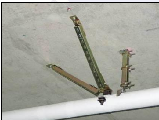
Lateral and vertical bracing for piping
