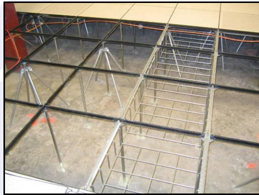
Raised-access floor bracing system
