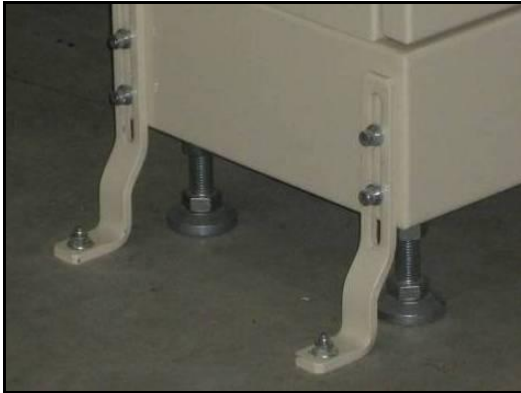
Floor-mounted manufacturing equipment anchorage
