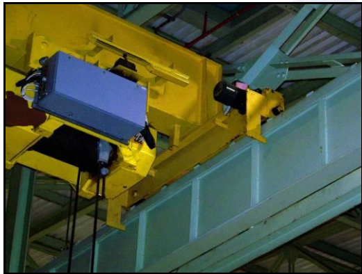
Bridge crane vertical restraint
